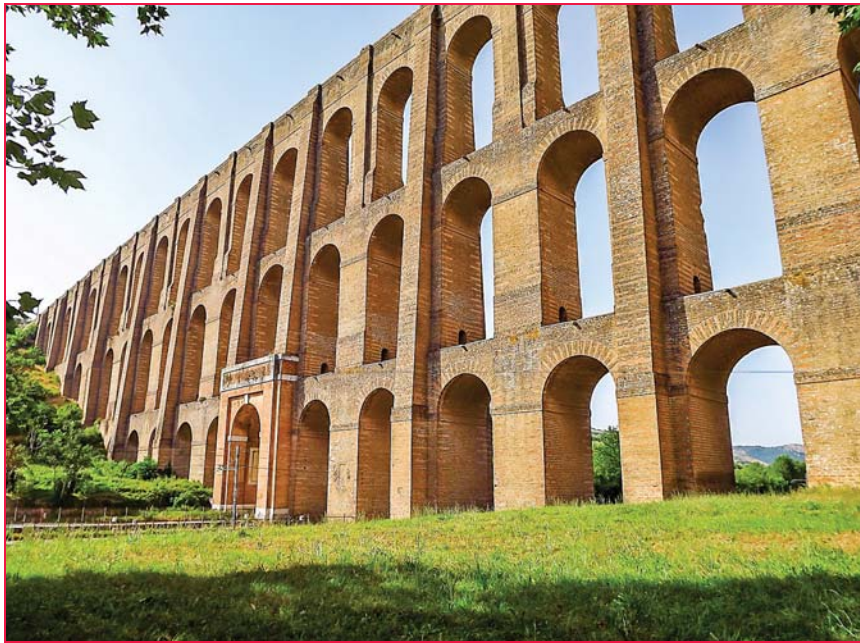
Figure 1a: Actual state of the Vanvitelli's masonry aqueduct
